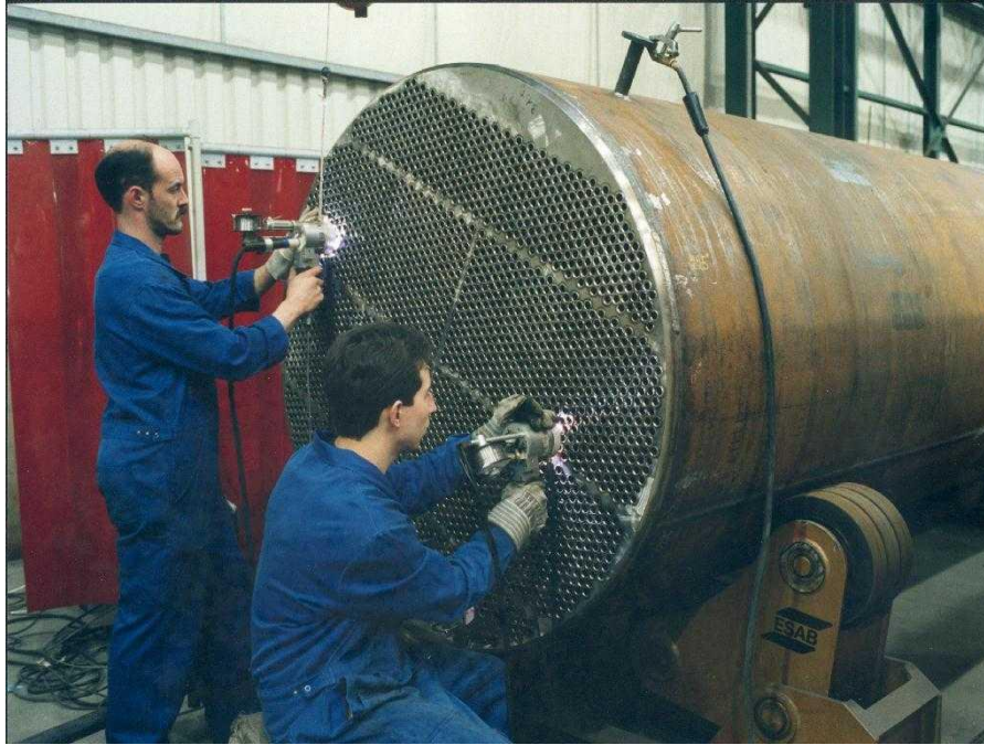
FIGURE 3 Heat Exchanger for VCM plant under construction.
