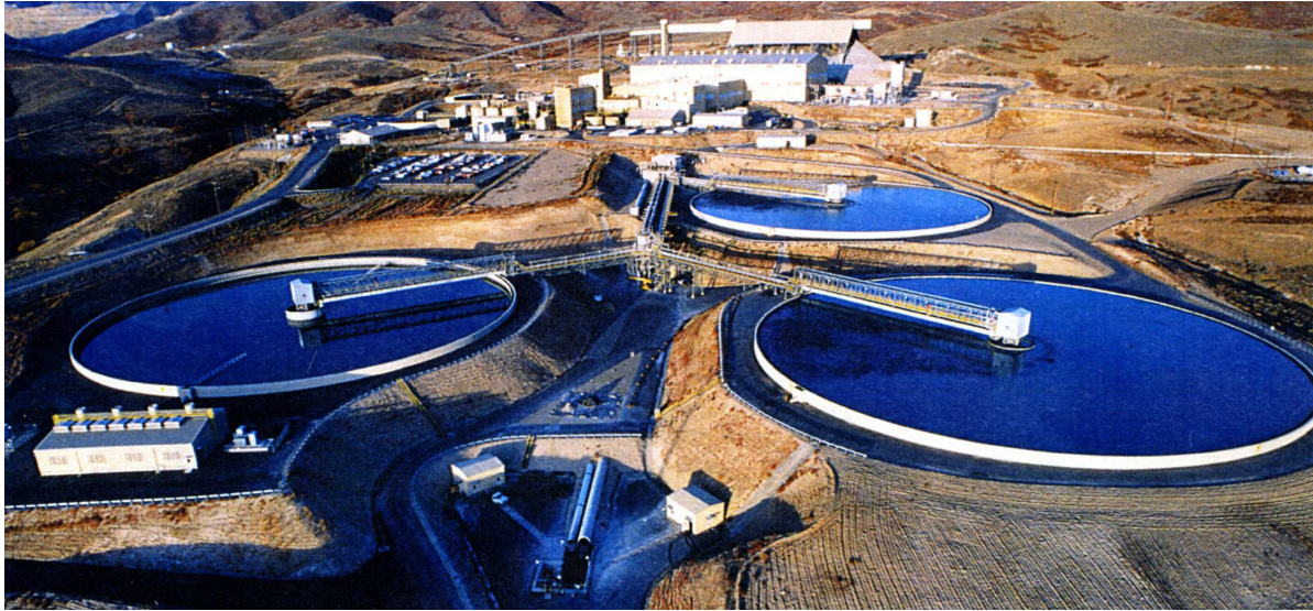
Figure 7 A typical thickener arrangement in an acid leach process. (Photo courtesy of F L Smidth)
